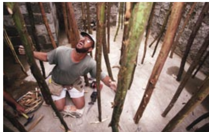
Tony Novak, CC St. Petersburg, sets saplings for the forms to pour concrete.
