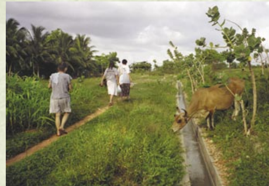
A cement channel runs from the mountain edge through a corn field to irrigate the fields and water the animals. It is also used for bathing.
